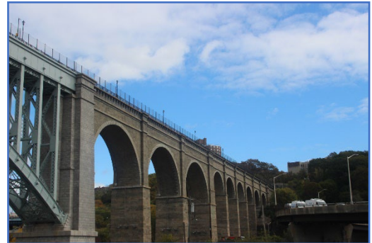
The Croton Aqueduct once crossed into Manhattan on this bridge.
